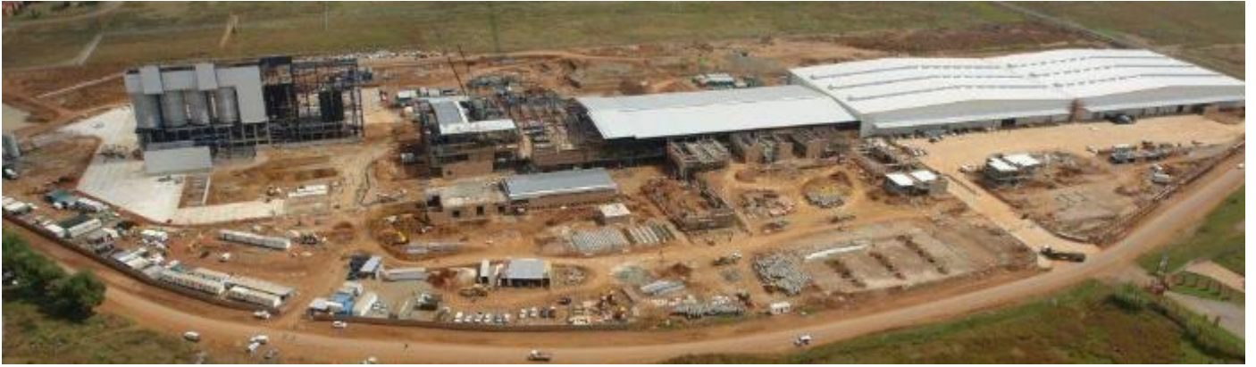
Consol Nigel site during construction
