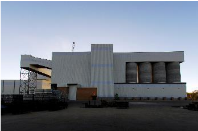
Consol Nigel Batch Plant on completion
