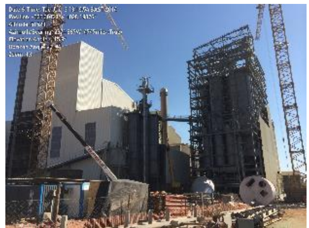
Batch Plant, Johannesburg
