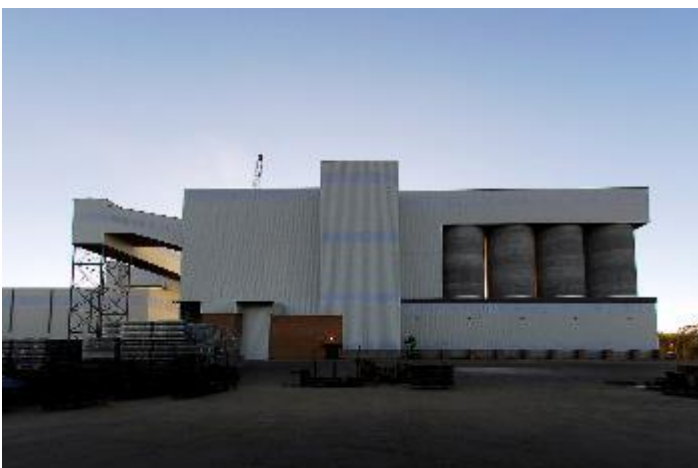
Consol Nigel Batch Plant on completion
