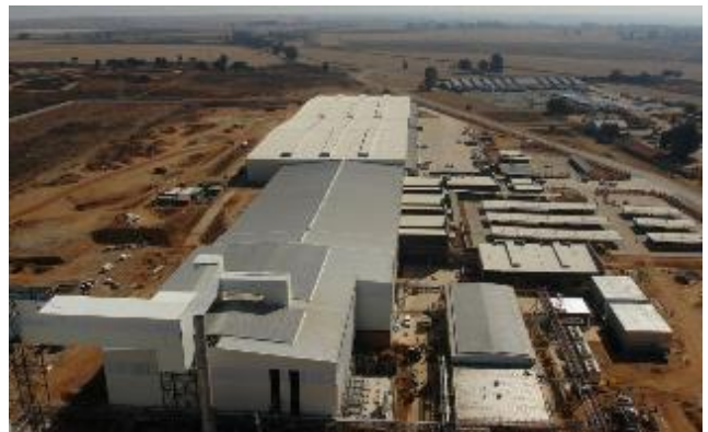
Consol Nigel Furnace Building & Warehouse
