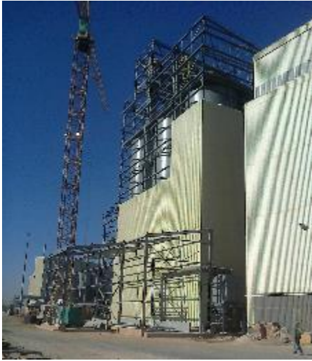
Batch Plant, Johannesburg
