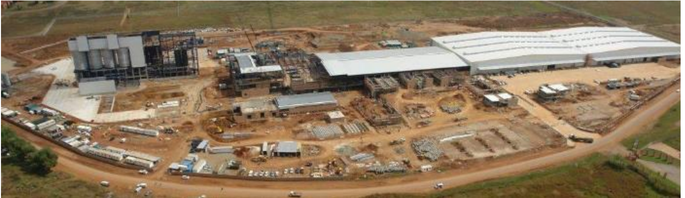
Consol Nigel site during construction
